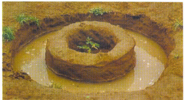
Rin Pit - Rainwater storage technique for Arid zone
