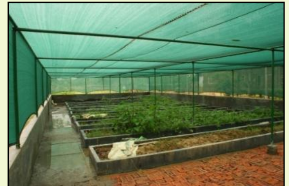
Under construction shade house
